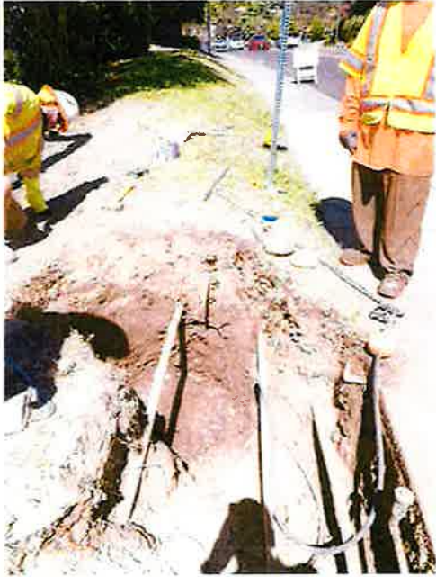
EXISTING BURIED MANHOLE PHOTO (1)
